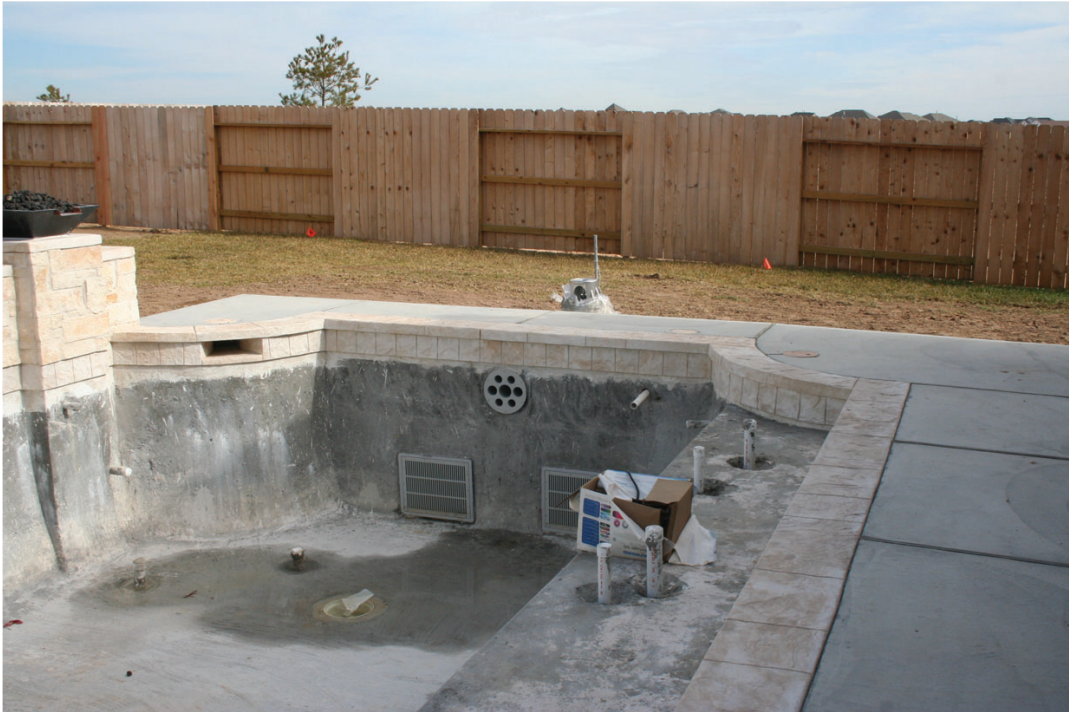
RIVERFLOW SWIMPOOL RETURN / DRAINS INSTALLED
